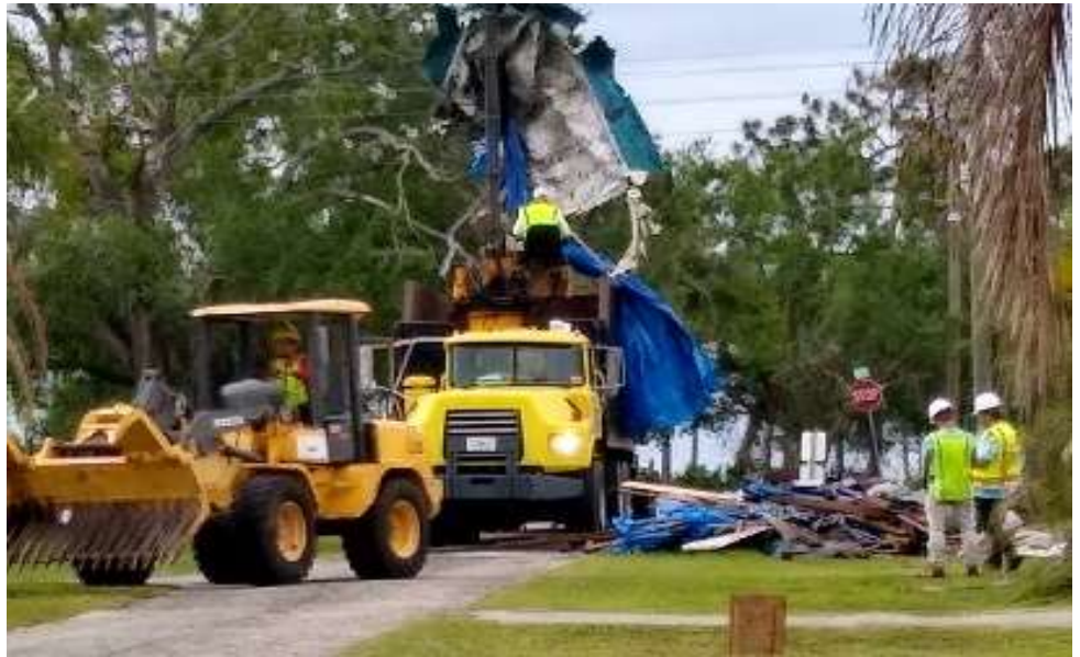
Florida Division of Emergency Management removing Debris on Indiana Drive
