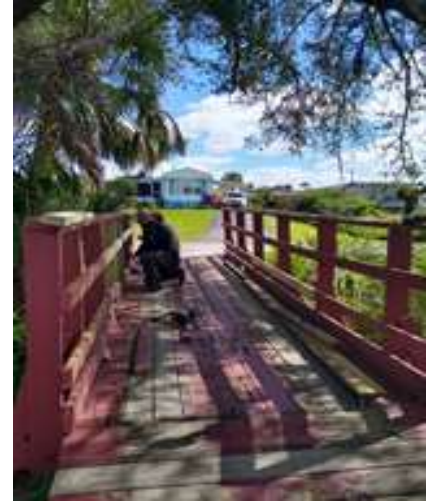
Larry Spurgin and Ken Kaprielian repairing the Michigan bridge
